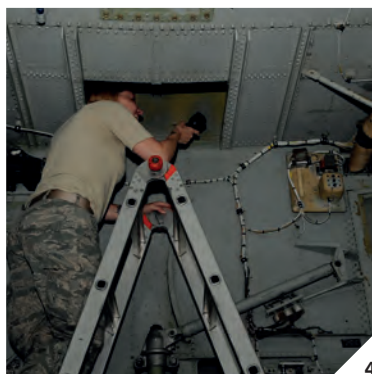
5 // A USN60 ultrasonic unit is used to detect cracks on the 694 bulkhead located in a crawl space above the B-52H bomb bay
